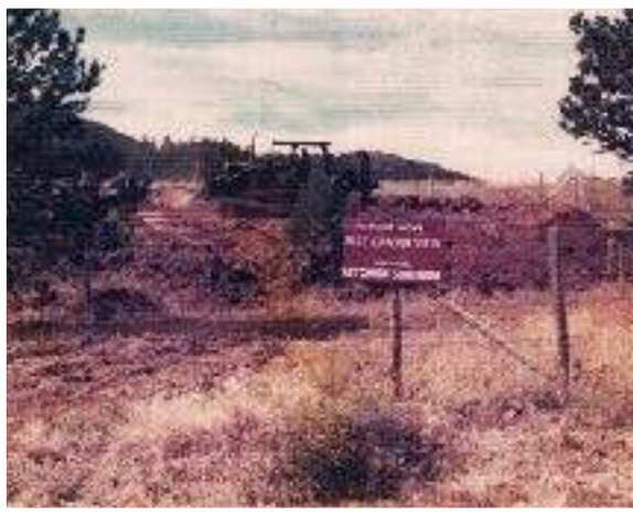
Grading for Station 1
